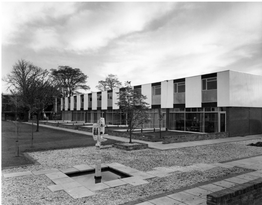
The eastern terrace in phase 1, photographed in 1964. RIBA Collections.
