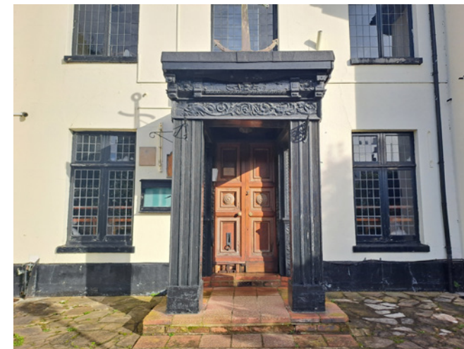
Classical motifs to the flat-roofed portico at the 19th-century Anchor Hotel on Church Square. The use of decorative moulding is unusually rich when compared to the restrained use of Classicism seen elsewhere in the Conservation Area. The age of the portico and its relationship to the original building is unclear, although it is visible in a photograph of the hotel from 1915. 02
