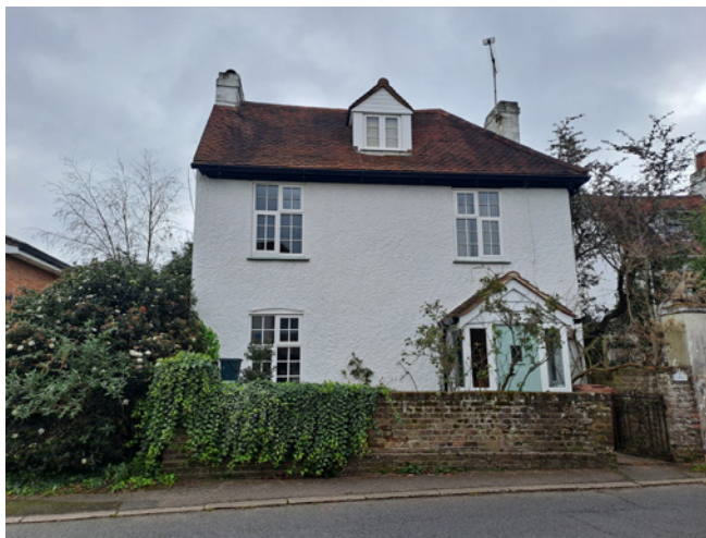
A low brick wall outside the historic property known as Rose Cottage on Upper Halliford Road.
