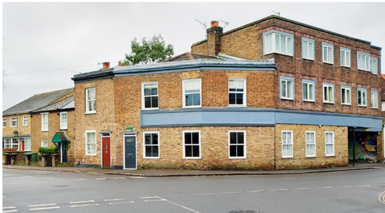
Evidence of a former shopfront at 22 High Street.
