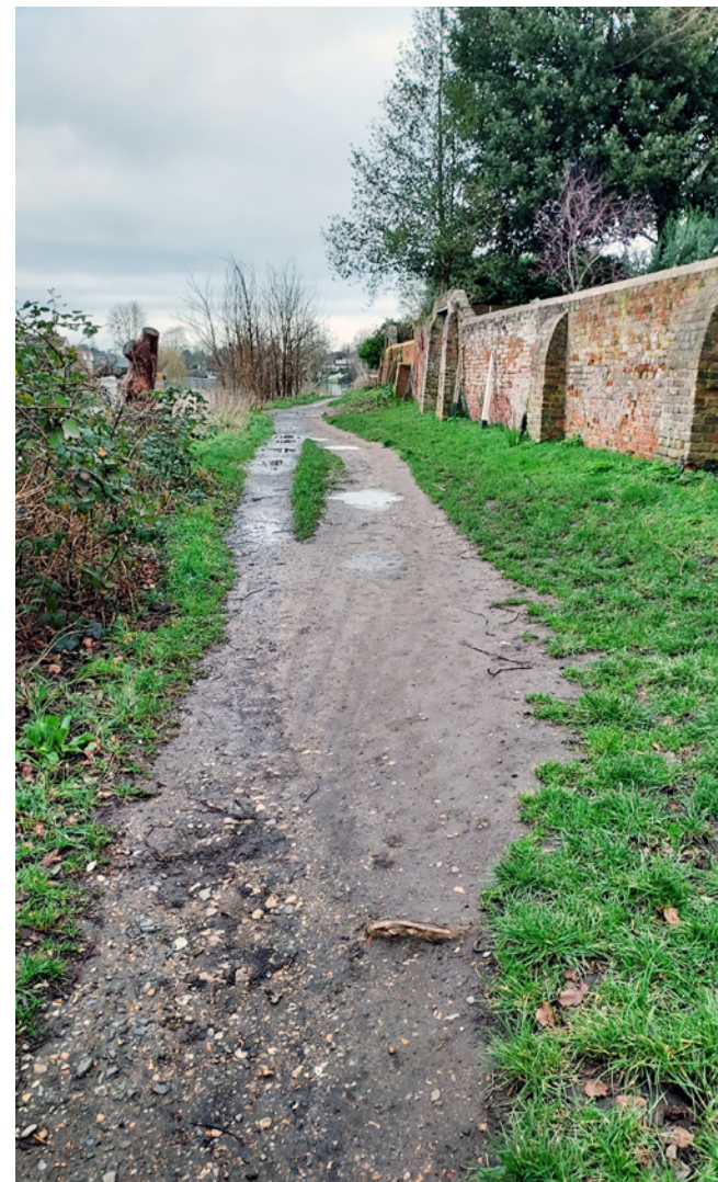
The listed brick wall along the northern portion of the Thames Side path
