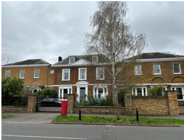
Hawke House, a Grade II listed early 18th-century building on the northern boundary of the Conservation Area. The right-hand wing was constructed in the late 18th century and the left-hand wing was added in the 20th century.
