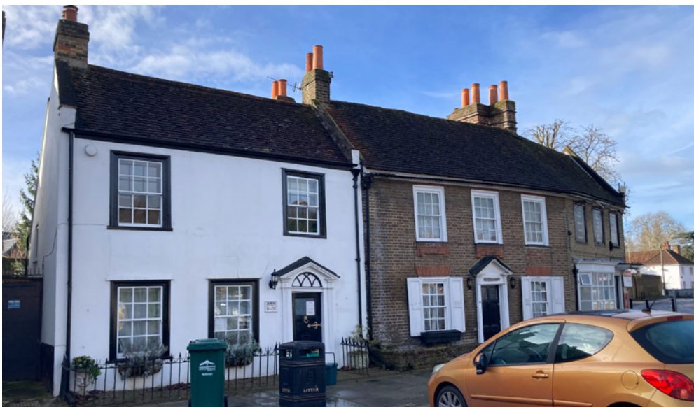
Historic timber-framed sash windows to the 18th century buildings on the south side of Church Square.
