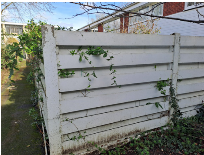
Plain, white-painted timber 'hit and miss' fencing in phase 3 of the estate.
