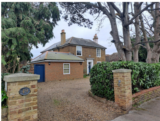
49 Upper Halliford Road. An 18th or early 19th-century dwelling with typical Georgian detailing including a square plan, regularly arranged sash windows and a small portico articulating the principal entrance.
