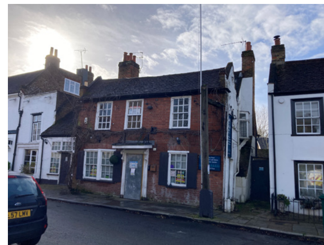
The Kings Head pub, currently vacant and in need of maintenance and repair
