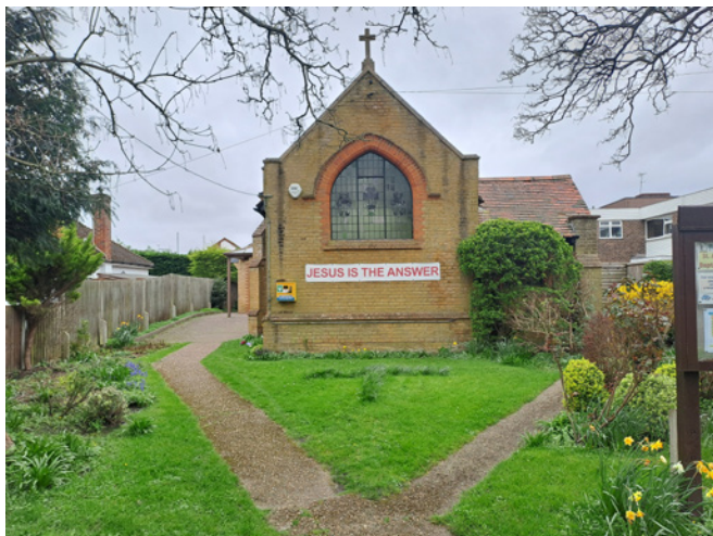
St Andrews Church, constructed in 1900, utilised a traditional materiality of exposed red and yellow brick.
