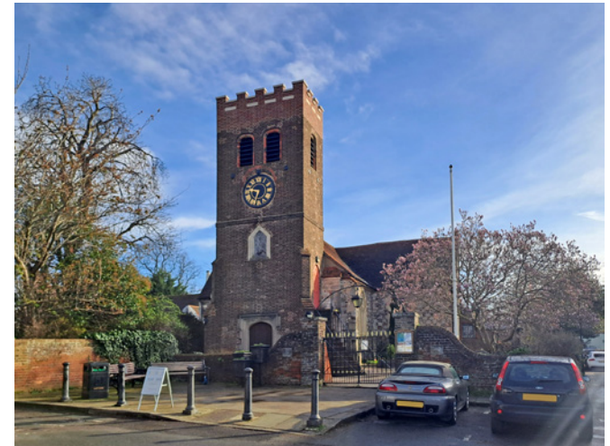
The distinctive brown brick tower of 1710, seen from Church Square.
