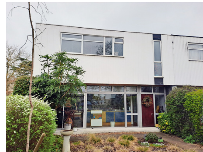
Original full-height glazing to the ground floor on an east-facing elevation in phase 1. The original plain door, faced with plywood, has been retained in-situ.
