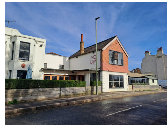
Hung clay tiles to a street-fronting elevation at the Red Lion, Russell Road.
