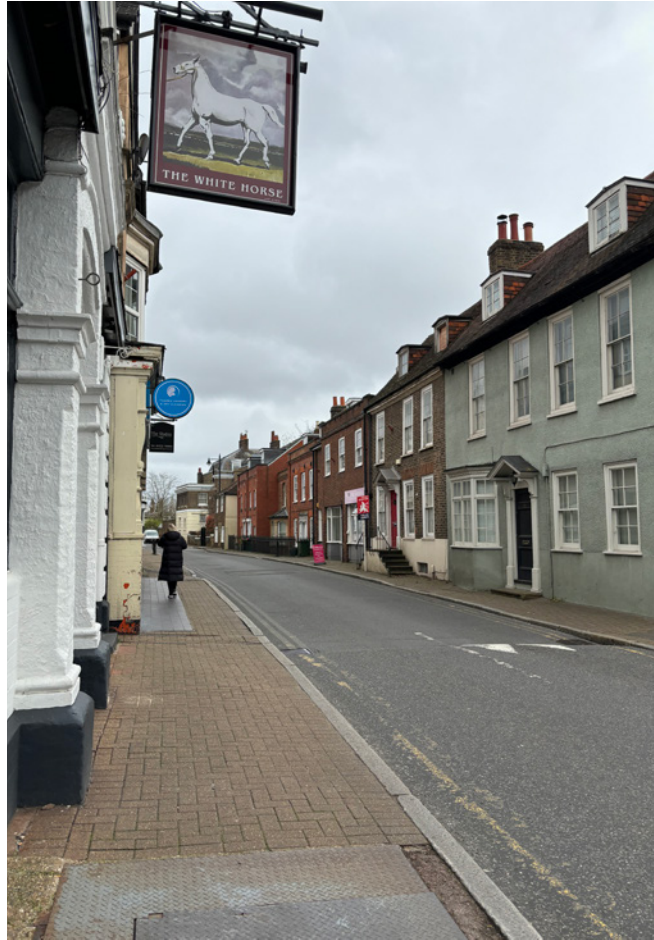
Looking east down Thames Street. Properties in this area generally front directly onto the public highway. The streetscape is characterised by the mixture of commercial and residential structures.
