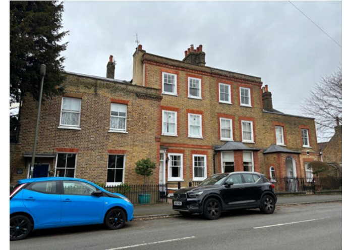
Moving further north, the historic properties are situated closer to the highway, creating a more enclosed character. This row of houses dates from the mid-late 18th century. In its use of exposed yellow/brown brick with red brick dressings, it mirrors 106 French Street slightly further south.
