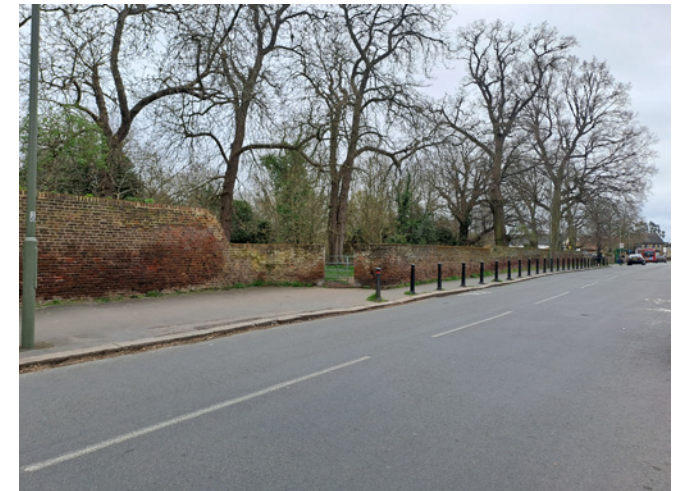
The red brick boundary wall on the eastern side of Green Street, beyond which lies Sunbury Park.
